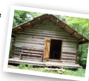
The original cabin fell into disrepair but its heritage is preserved. It was reconstructed using wood from a 1910 area building and nearby logs. Using a broad axe, the logs were faced on two sides and stacked with the rounded sides adjoining, mirroring the construction techniques of the 1930s. The dovetailing of corners helped to secure the logs and shed water. Some modifications have been made to the original design to increase the life of the cabin.
